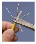
2) Remove center spline as close to jacket end as possible.
