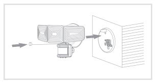
6 Using silicone caulking compound, caulk completely around where the light fixture meets the wall surface to prevent water from seeping into the outlet box.
